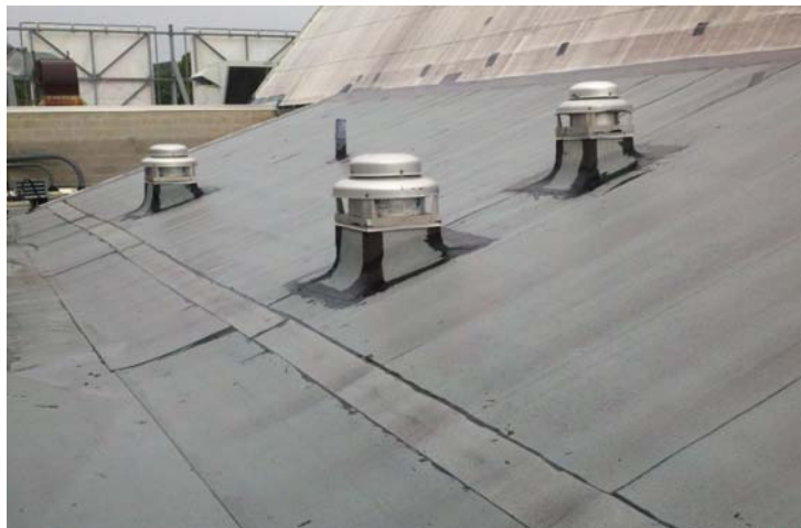
3: Roof mounted exhaust fans
