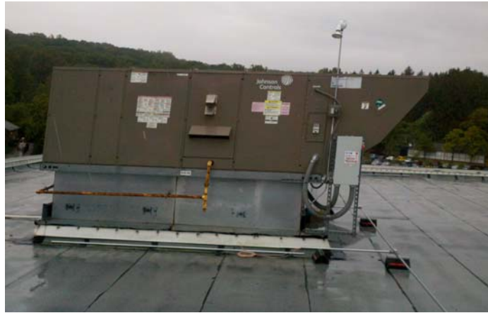
5: Rooftop unit RTU
